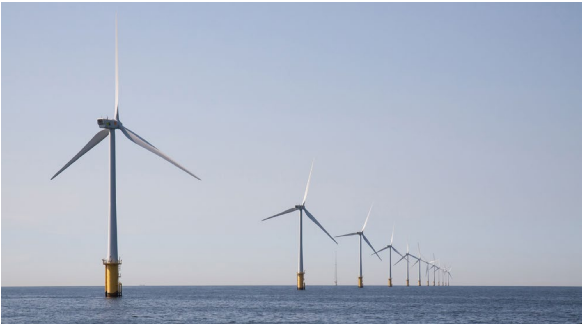
Offshore wind farm
